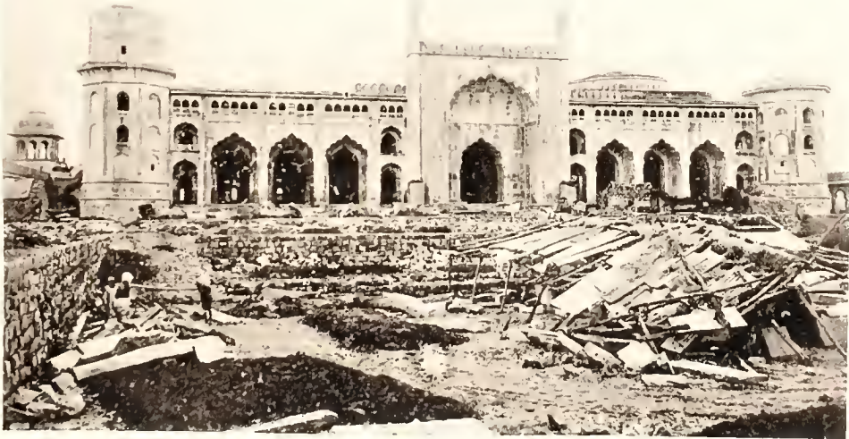
MOSQUE NOW UNDER CONSTRUCTION, BHOPAL
